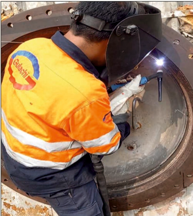
Tig welding of manway
