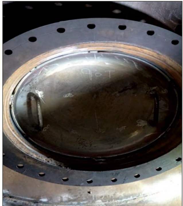
Fit up after welding.
