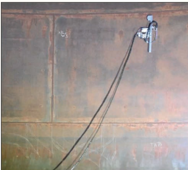
Corrosion mapping test
