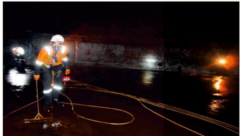
Airline masks used for continuous respiration along with PPE dress to avoid possible skin contact with ammonia vapour
