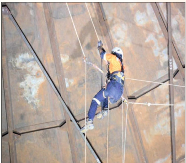
Roof inspection using Rope Access gears.
